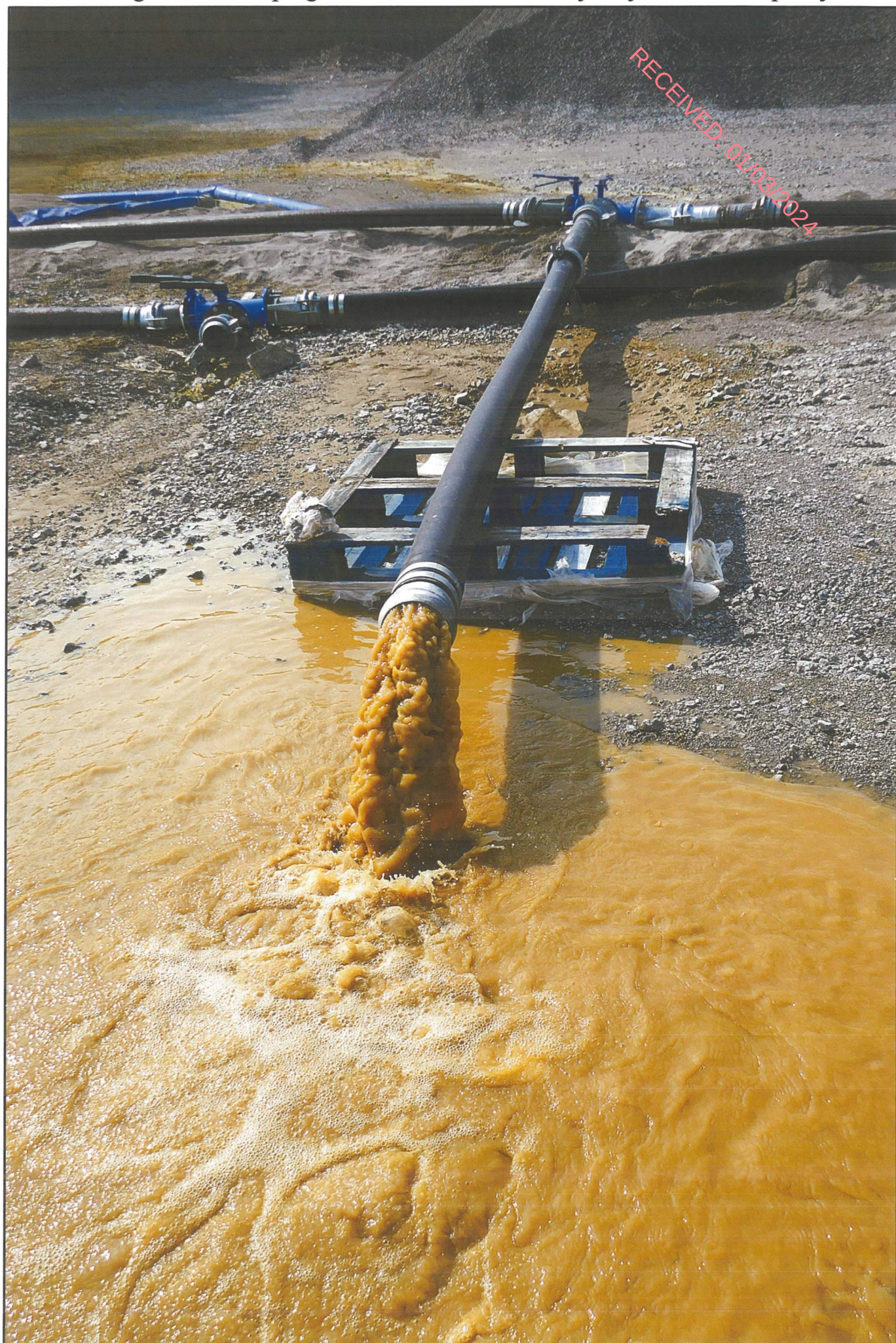
Figure 3.3 Pumping initial water with a heavy clay load to the quarry floor
