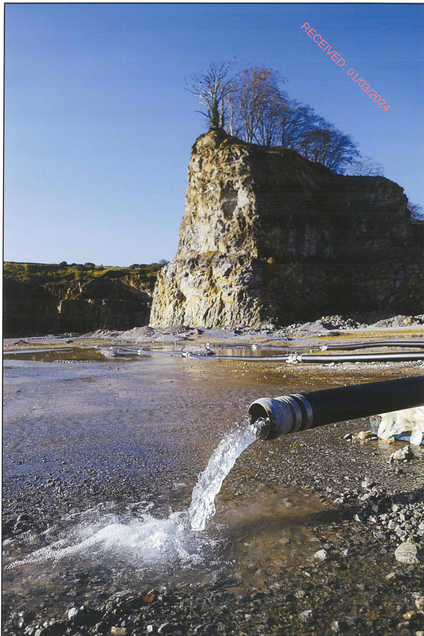
Figure 3.4 Clear water discharge before diverting the flow direct to the settlement pond
